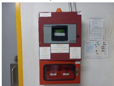
Fire Alarm Control Panel
