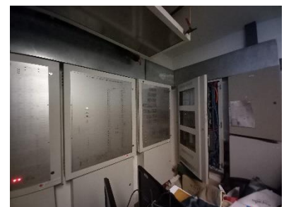
Graphic Annunciator Fire Alarm System
